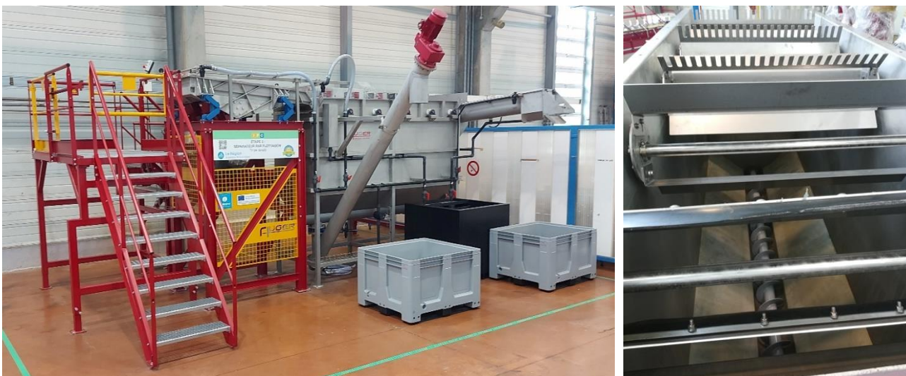
Figure 14: Dynamic flotation bath (left: outside view, right: inside view)
